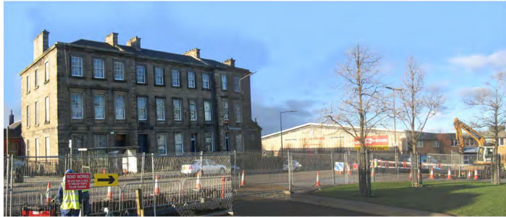
existing listed building adjacent to site
