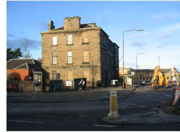
6. view of corner of site at granton square
