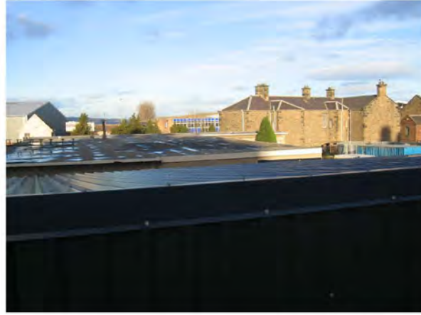
5. view from west granton road across site
